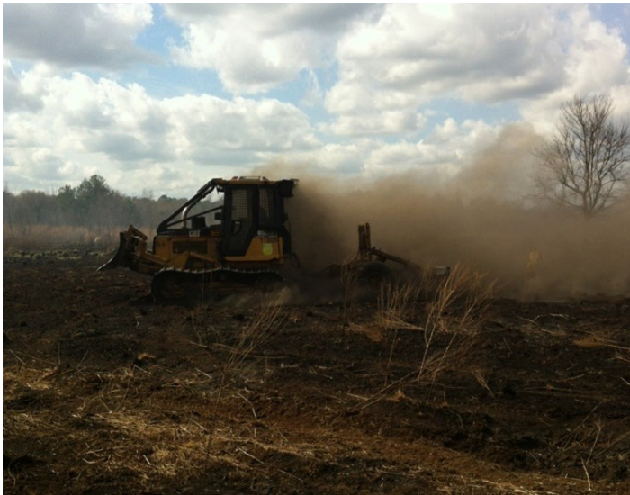
Figure 1. At the Olive Fire (Levy Prairie, Putnam County, Florida), many passes of this bulldozer were required to cut a fireline to mineral soil through the thick muck.
